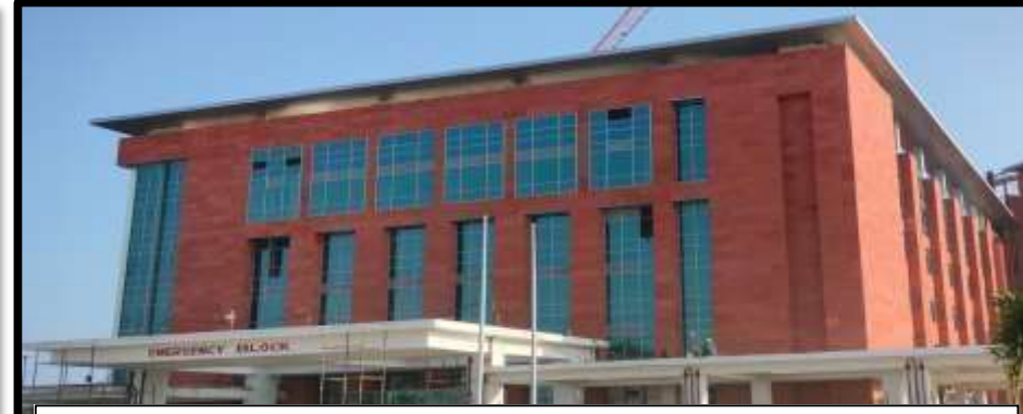
HOSPITAL TOWER – 2, Emergency Block (B+G+4)
